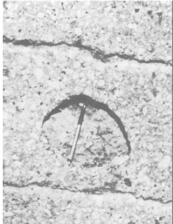
Figure 5-7. Small spall.
