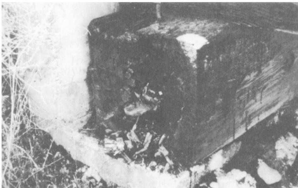
Figure 5-14. Advanced wood decay in crosstie.
