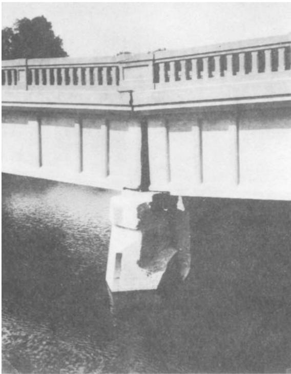
Figure 5-22. Movement due to scour.
