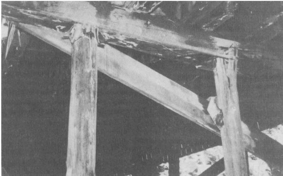
Figure 5-15. Advanced wood decay in bent cap.
