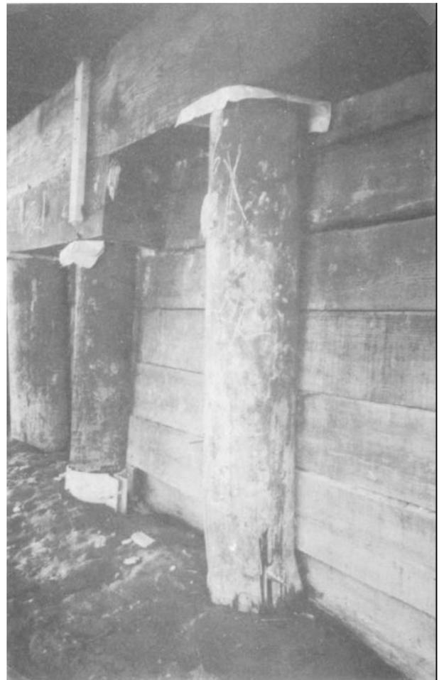
Figure 5-17. Buckled timber pile due to overload.
