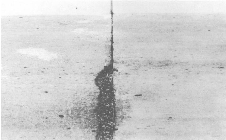
Figure 5-11. Joint spall.
