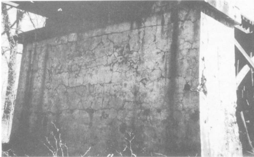
Figure 5-1. Pattern or map cracking on a pier.
