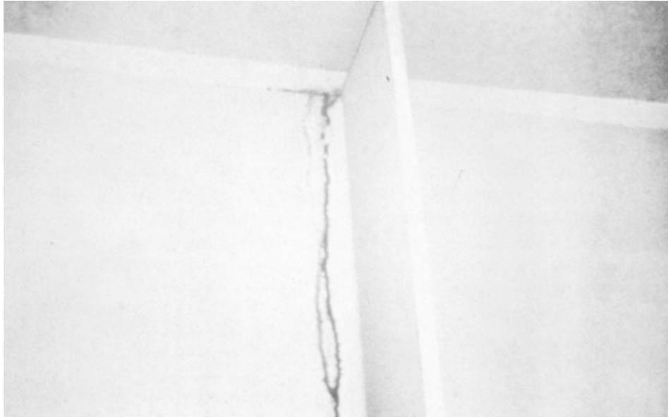
Figure 5-12. Rust stained crack in steel girder.
